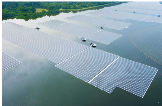
Floating solar PV system on Tengeh Reservoir
