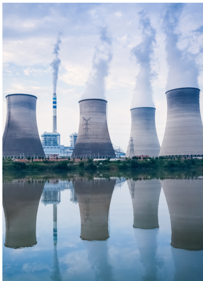
Coal-fired power plant, cooling towers and river surface reflection, Jiangxi, China
